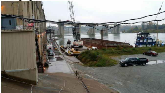
Dredging at Falls of Ohio Power Station
